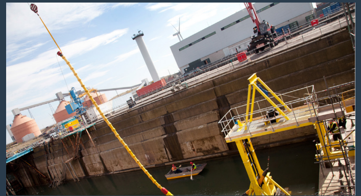
Tekmar's TekLink system in testing at the Catapult's National Renewable Energy Centre in Blyth, Northumberland.
