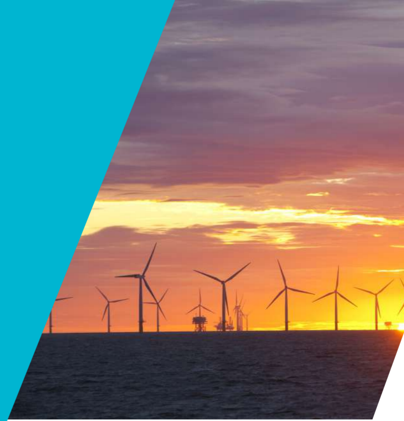
Image ^ Burbo Bank Offshore Wind Farm Credit: Ørsted
